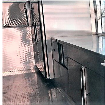
Equipment sealed to each other, floor, and back wall to prevent debris from accumulating underneath, behind and between equipment.
